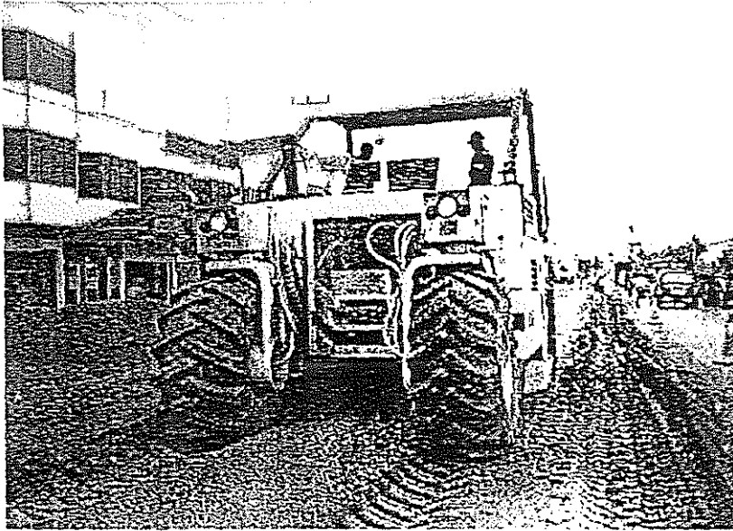
Gambar D.3 - Pencampuran kering ( dry mixing )
