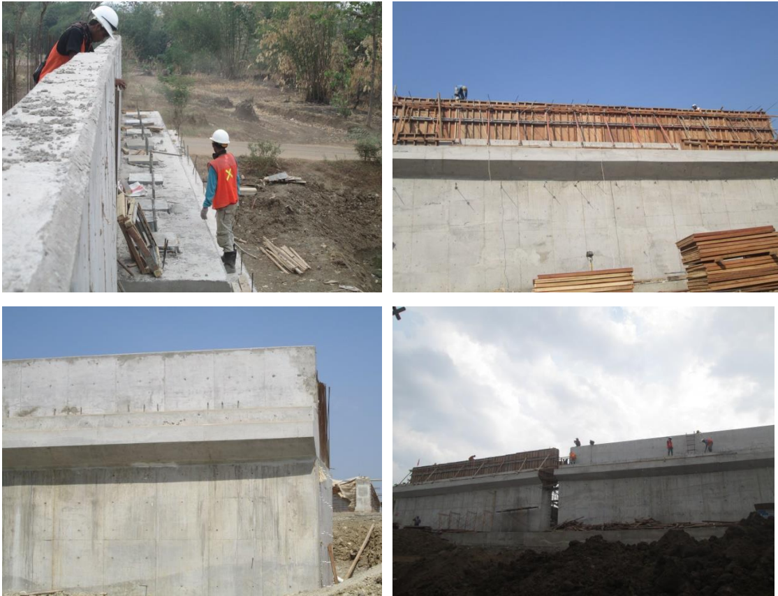
Gambar 5.16 - Pekerjaan finishing abutment
