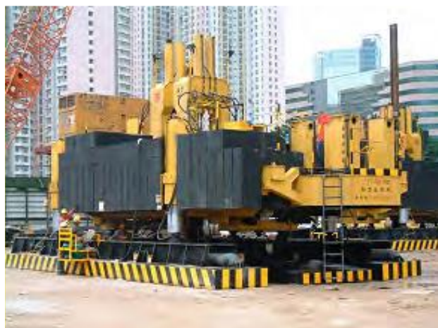
Gambar 4.17 - Mesin penekan hidrolik ( jacking ) (Geo Publication, 2006)
