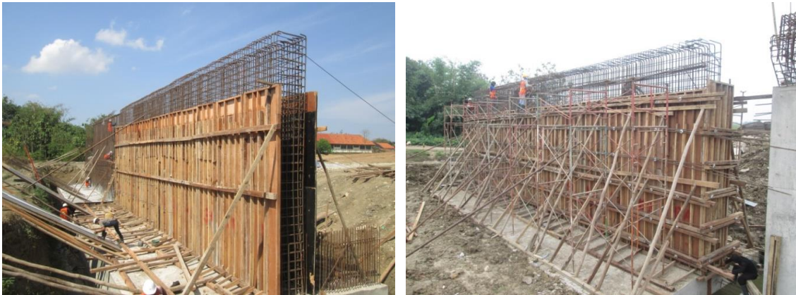
Gambar 5.13 - Pekerjaan bekisting badan abutment
