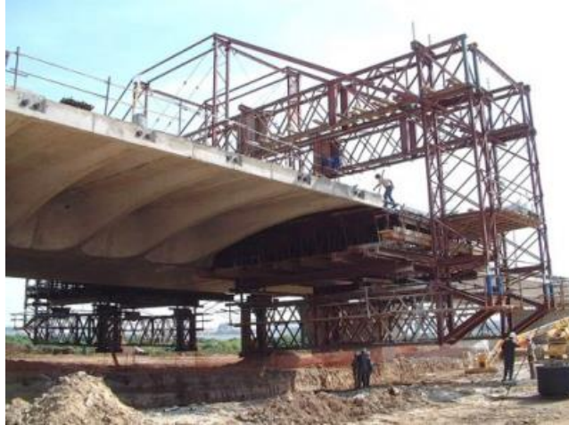
Gambar 3.20 – Perancah travelling
