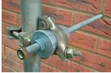
Gambar 3.15 – Angukur ( anchorage )
