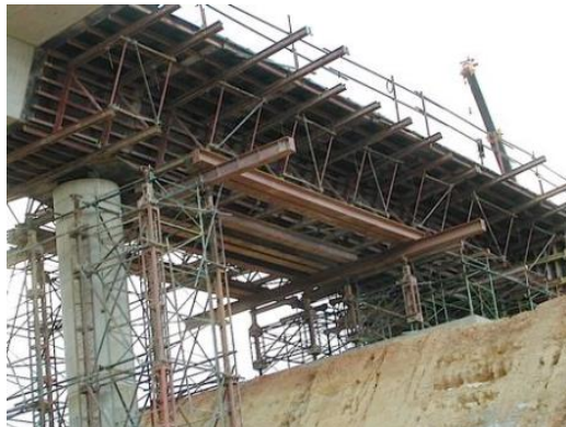
Gambar 3.16 – Perancah penopang jembatan ( bridge shoring )
