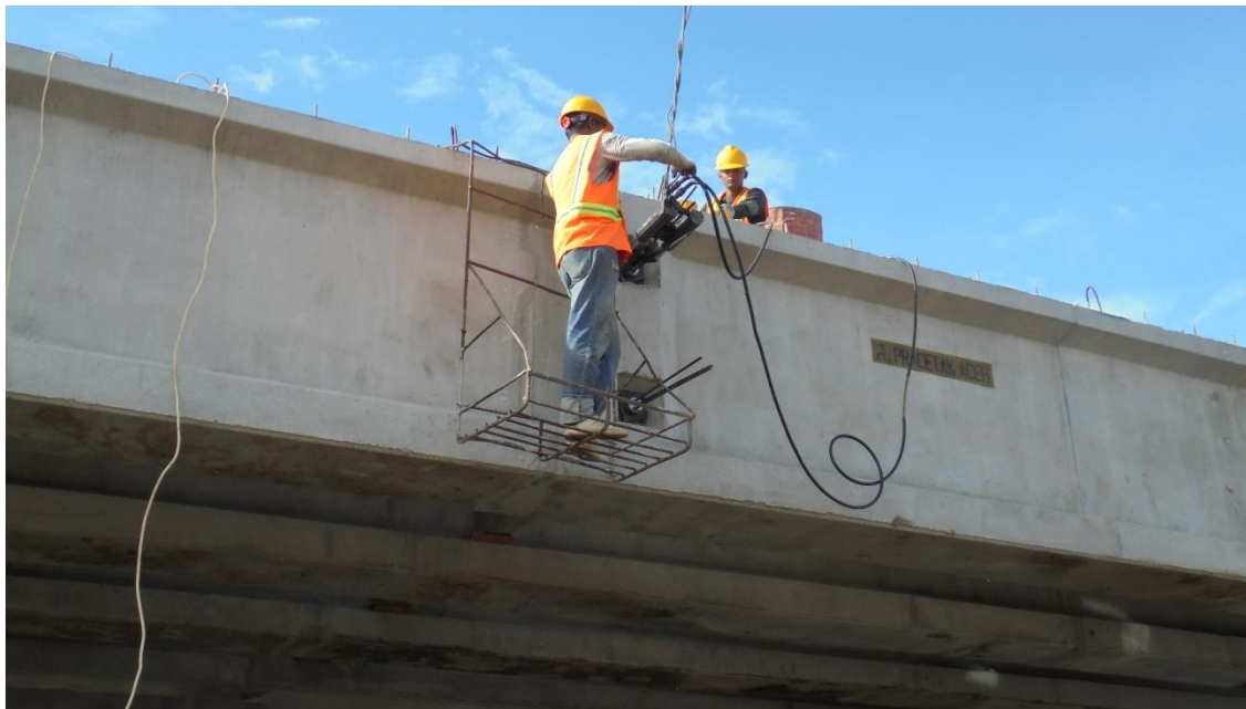
Gambar 6.37 - Stressing Lateral
