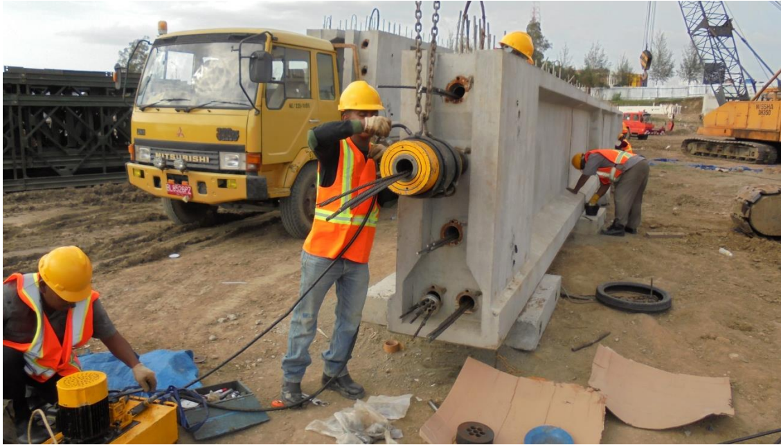
Gambar 6.21 - Persiapan stressing Gelagar
