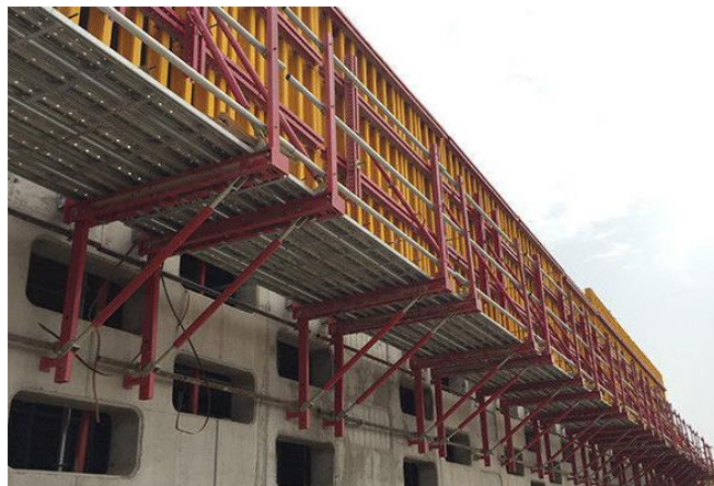
Gambar 3.10 – Perancah tupang siku ( cantilevered scaffolding )
