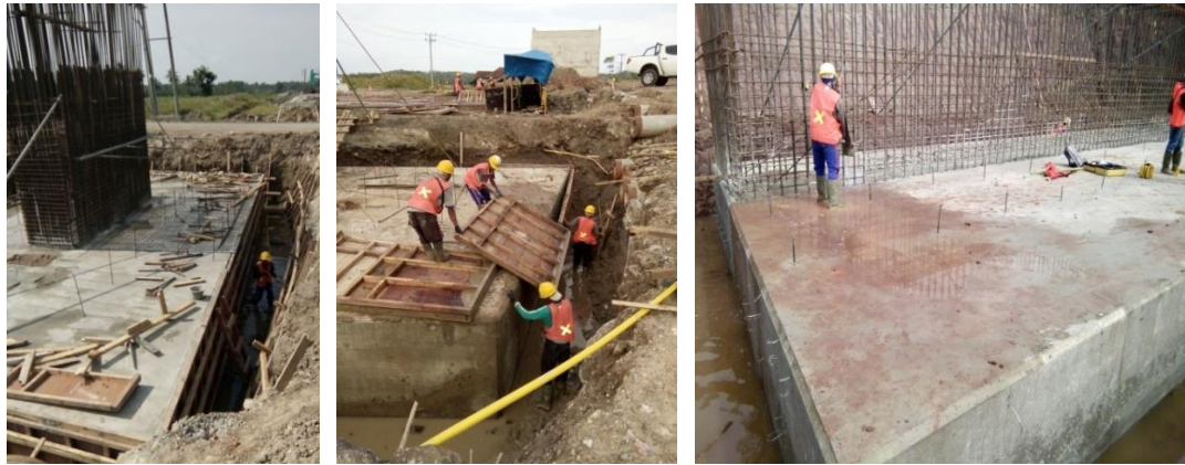
Gambar 5.24 - Pekerjaan finishing poer ( pile cap )
