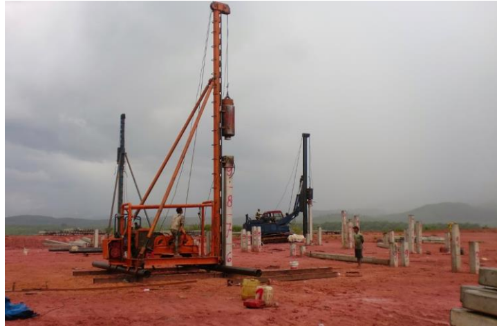
Gambar 4.14 - Drop hammer
