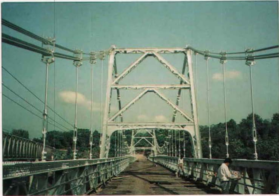
Figure A4.21 - Superstructure Type TBI Suspension Bridge
