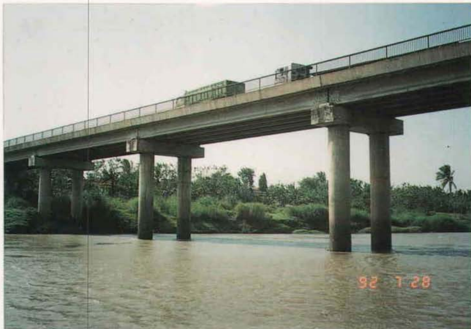
Figure A4.15 - Pier Type D Two Column
