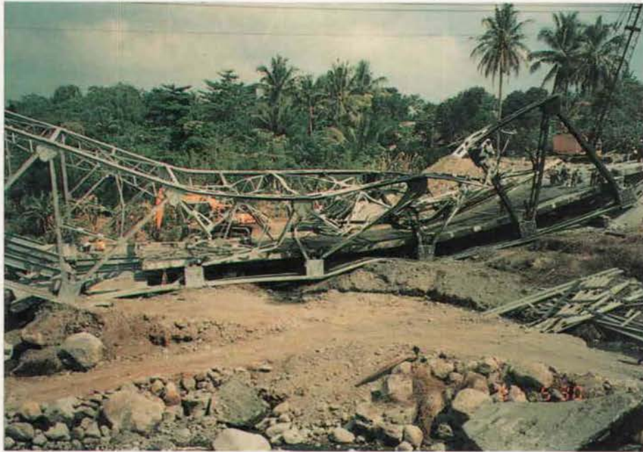
Figure A4.91 - Bridge collapsed due to fire
