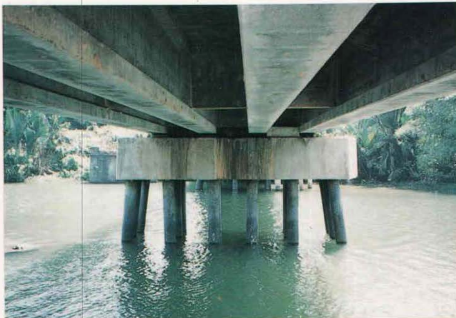
Figure A4.12 - Pier Type C Pile Cap
