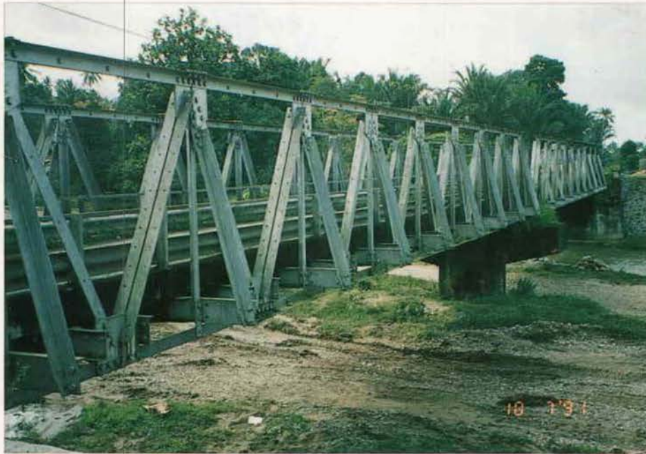
Figure A4.44 - Superstructure Type RBU Callender Hamilton Steel Truss (Type C)
