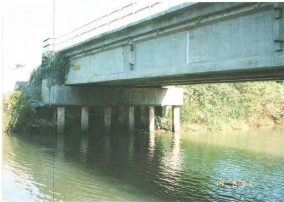
Figure A4.5 - Foundation Type T Driven Pile
