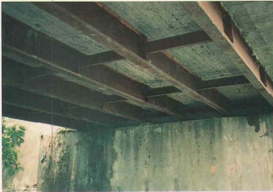
Figure A4.25 - Superstructure Type GBI Indonesian Steel Girder (Painted)
