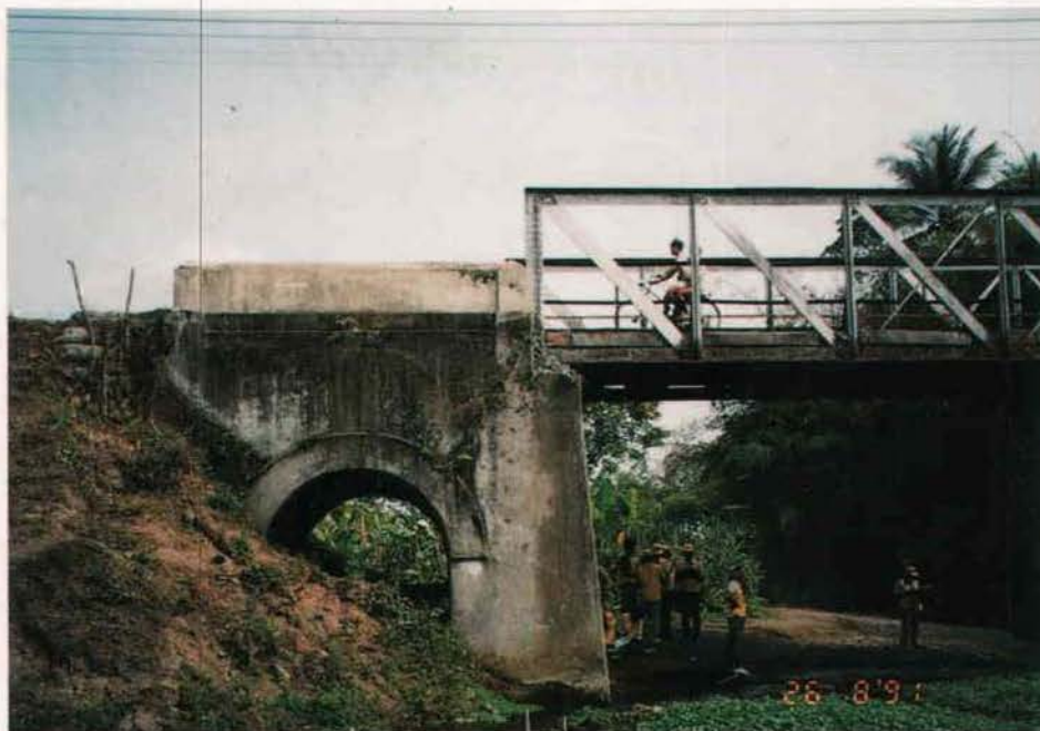
Figure A4.11 - Abutment Type K Special Abutment
