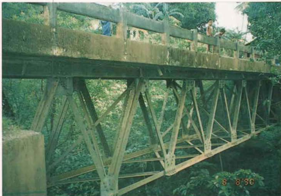
Figure A4.47 - Superstructure Type RBU Callender Hamilton Steel Truss (Deck Type)
